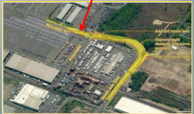
North Ave. / McLester St. Curve Realignment Completed - 12/11
